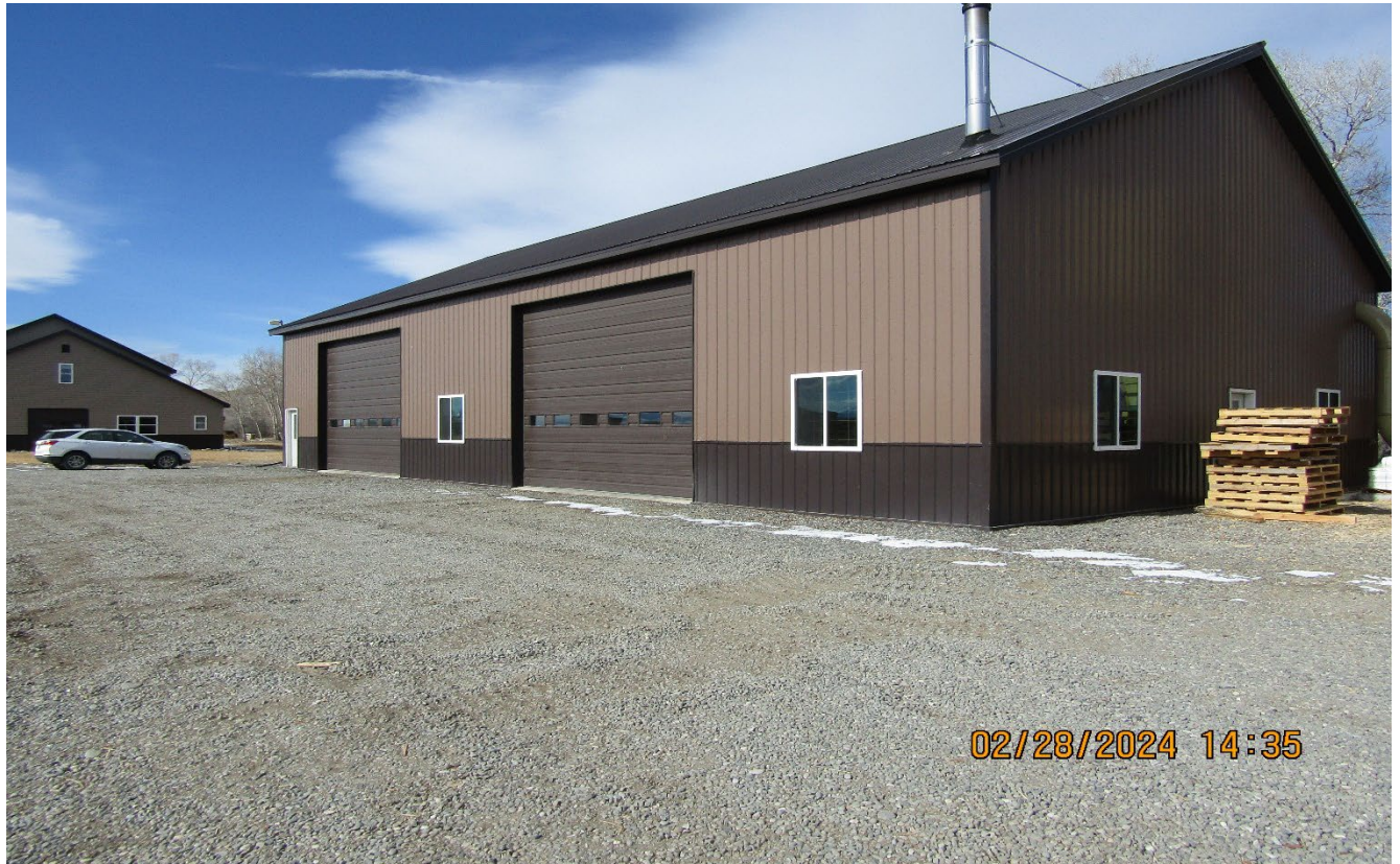
497 Photo 3: Structure for Use. Photographer facing Northwest.
