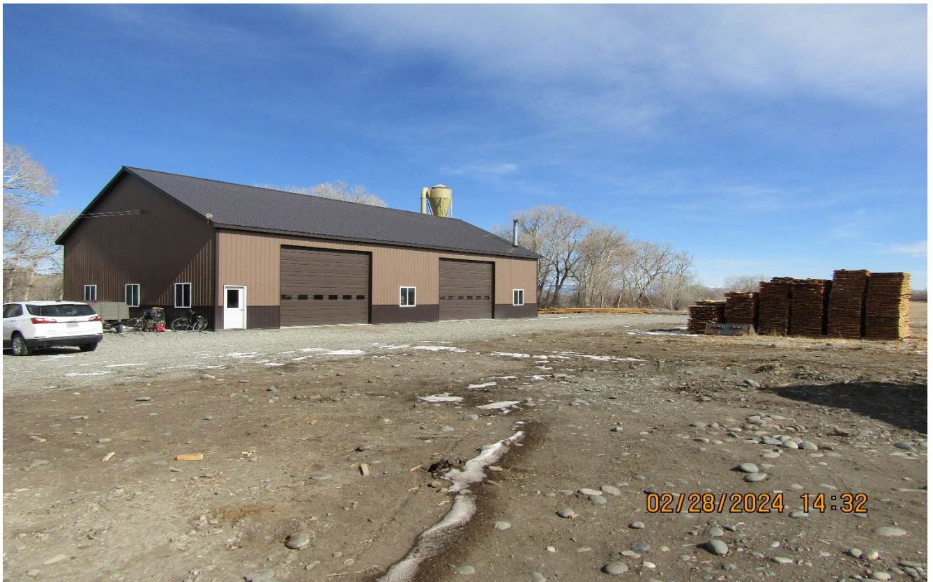
496 Photo 2: Structure for Use. Photographer facing Northeast.
