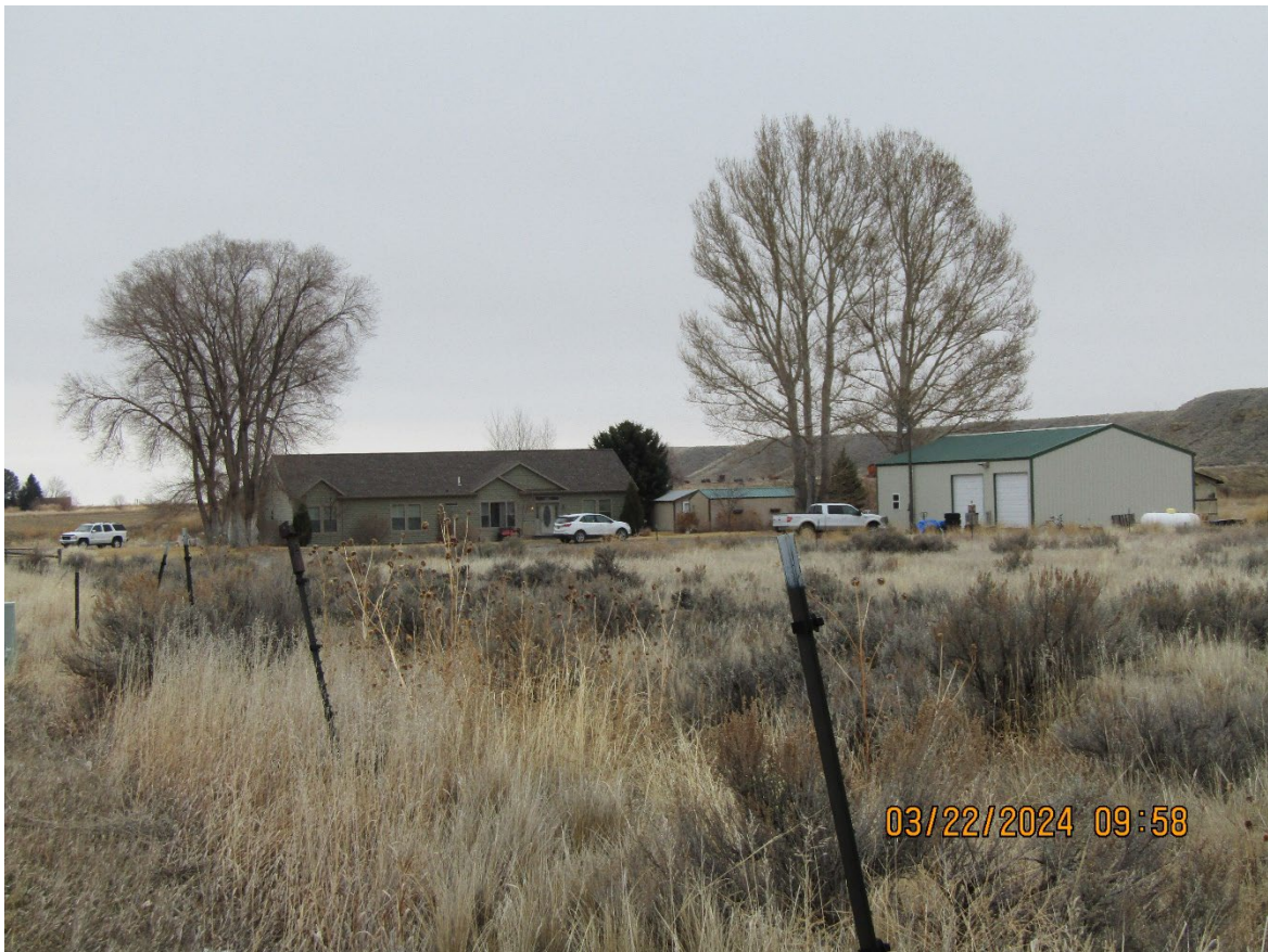
830 Photo 7: From the north boundary of proposed Lot 4, facing southeast across the 831 lot to view the existing development.
