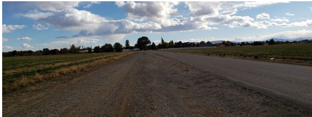
Looking south, near Lane 8
